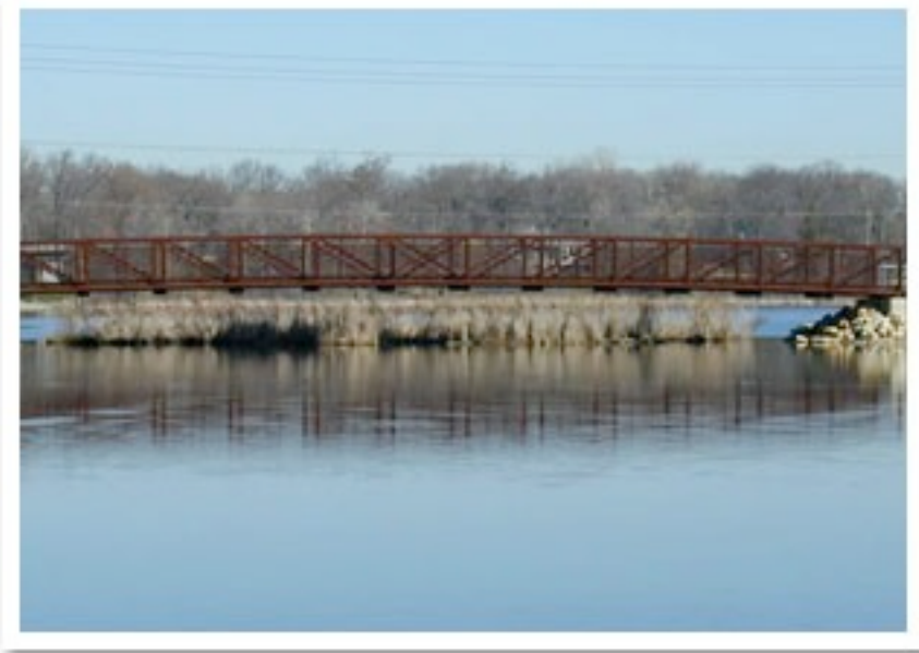
1997: New Luce Line bridge installed
